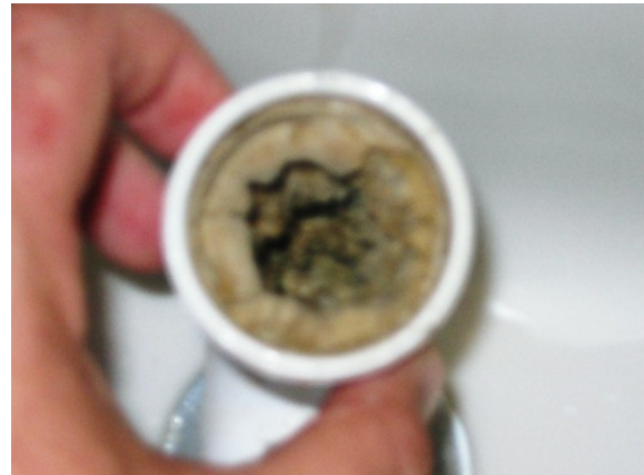
The pipe-work whilst using PDCB BLOCKS
